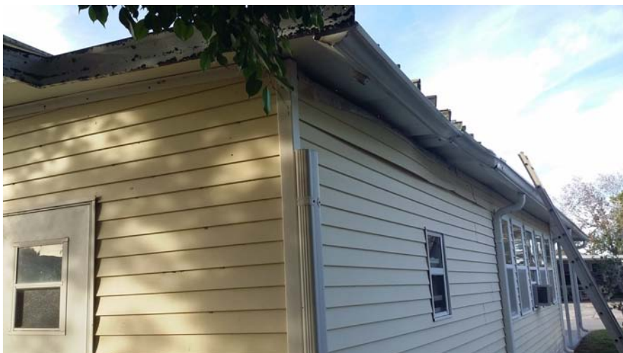
571 Dolphin (rear). Fascia/shed/siding damage.
