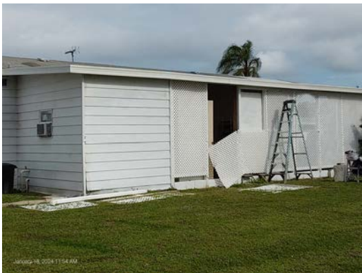
526 Persimmon Lattice in need of repair. 01/19/2024
