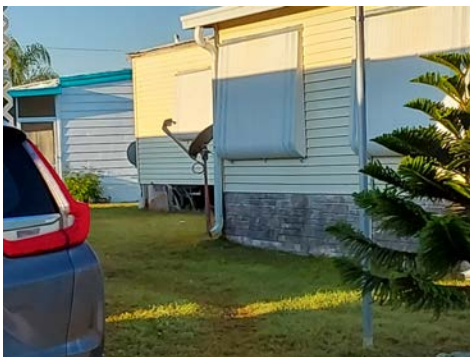
951 Frangi Pani Dr. Skirting needs to be replaced / repaired. 01/19/2023
