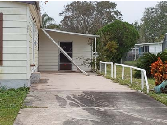
909 Hemlock St. Exterior maintenance: Roof / screen door damage, needs to be repaired. 12/12/2022
