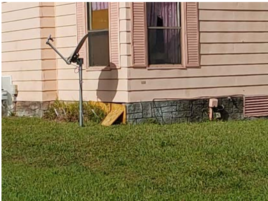
506 papaya Skirting needs to be replaced / repaired. 12/28/2022
