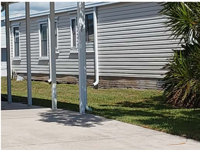
519 Sapote Skirting needs to be replaced / repaired Aug 25, 2022
