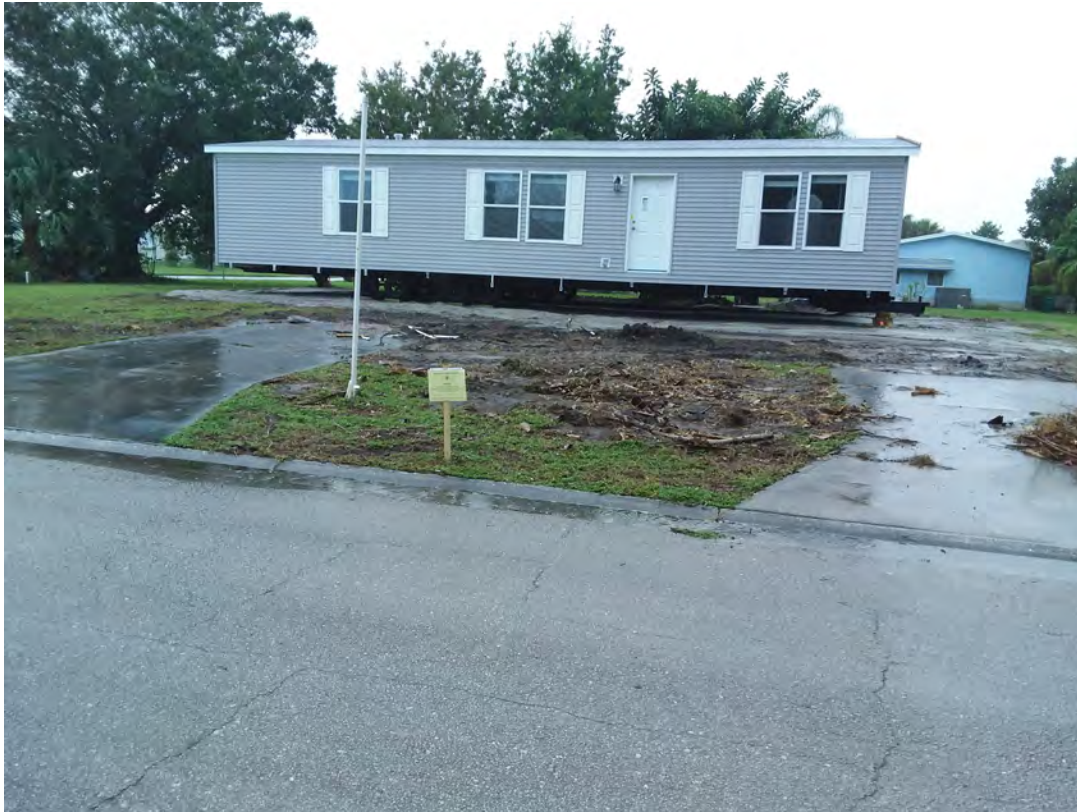
Photo: 398 Egret. Posted notice. STOP WORK.
