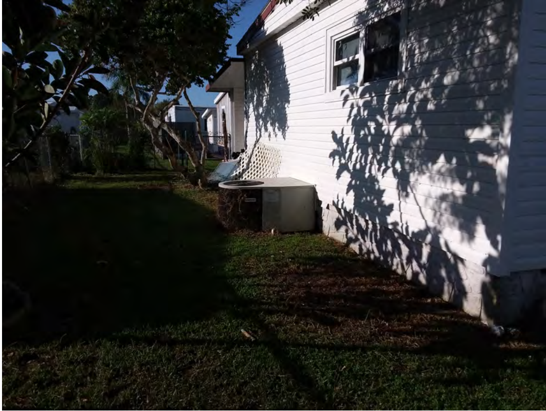
Photo: 915 Wren.Unapproved items - Debris
