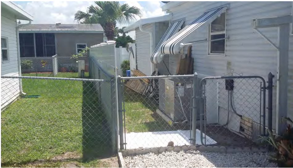
481 Marlin. Unapproved privacy fence. Left side. Peter Essig Jun 10, 2018
