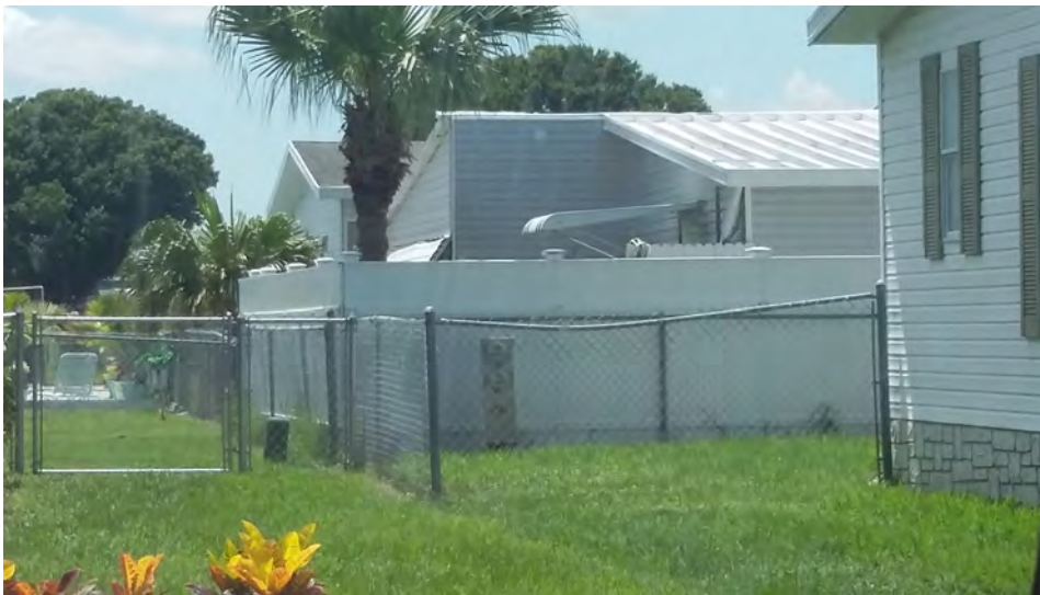
481 Marlin. Rear. Unapproved privacy fence. Peter Essig Jun 10, 2018
