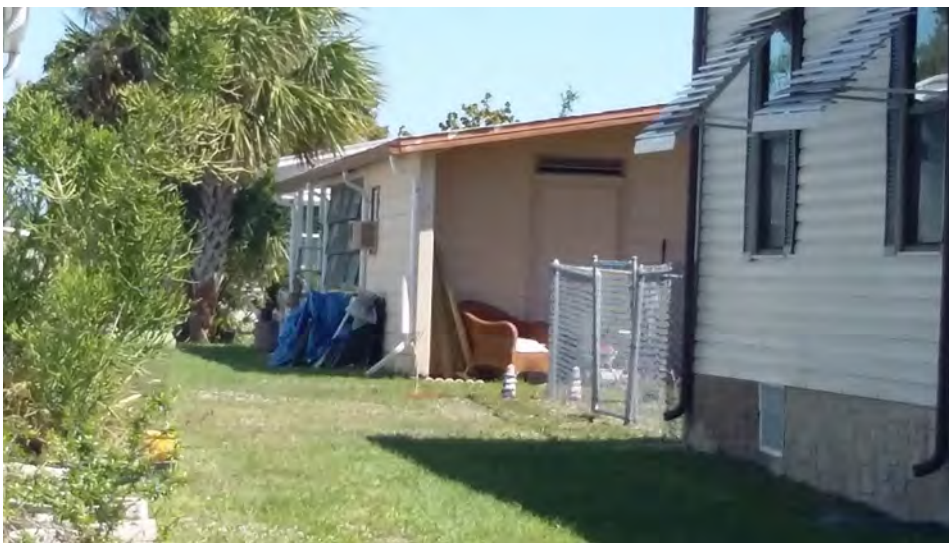
707 Periwinkle. Unapproved items around carport sides and rear of the house. Mary Barry Mar 07, 2019
