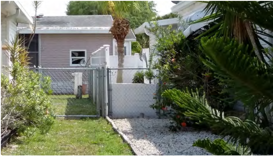
481 Marlin. Post-VC re-inspection. Too much privacy material. Peter Essig Apr 06, 2019
