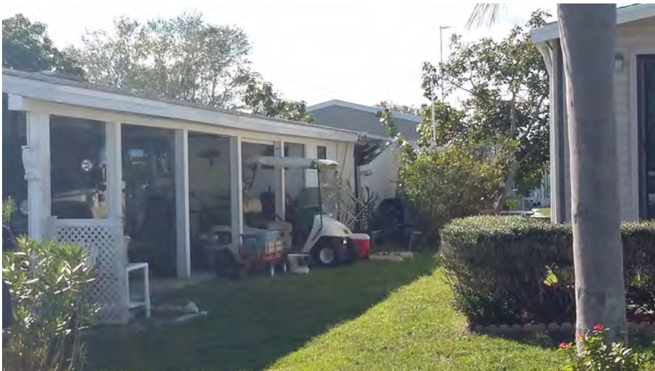
709 Wedelia. Roof/fascia damage. Peter Essig
