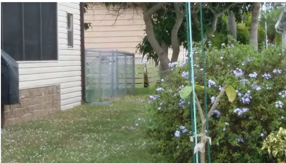
707 Periwinkle. Unauthorized items/debris in lawn; unapproved pallet fence on rear of property. Peter Essig Nov 20, 2018
