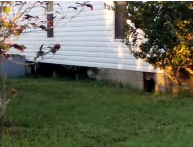
947 Jacaranda. Skirting needs to be repaired / Replaced. ARCC permit required. Mar 02, 2020
