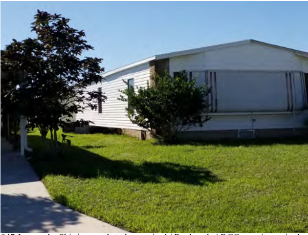
947 Jacaranda. Skirting needs to be repaired / Replaced. ARCC permit required. Jan 07, 2020
