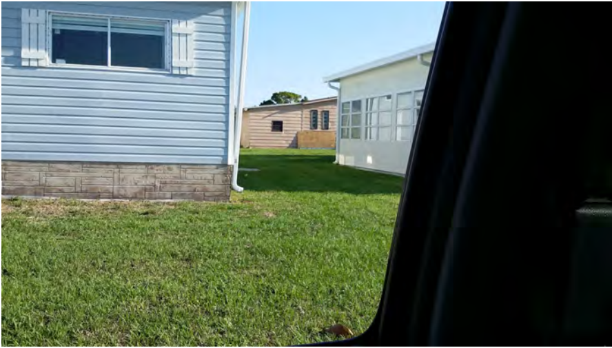
516 Egret (rear). Post-VC re-inspection. Unapproved item(s)/debris. Peter Essig May 16, 2019
