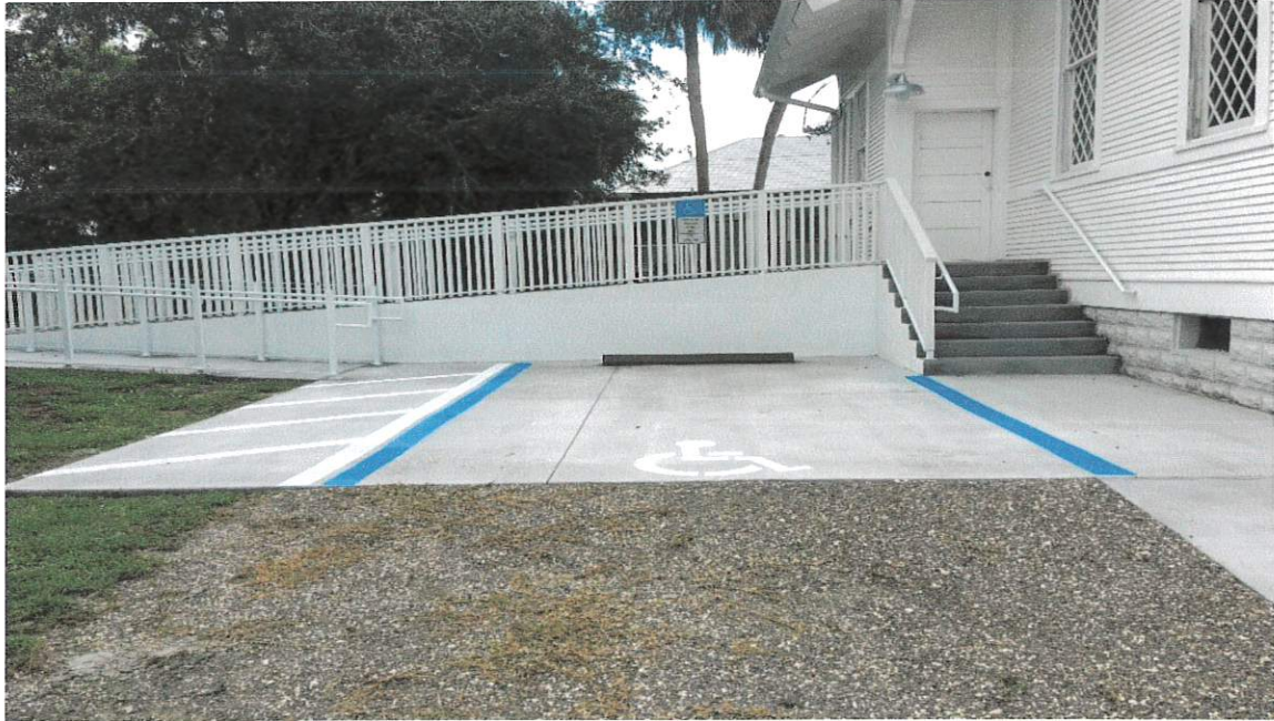
Picture #1: ADA Ramp, Stairs, Aluminum Rail w/ Wood Pickets
