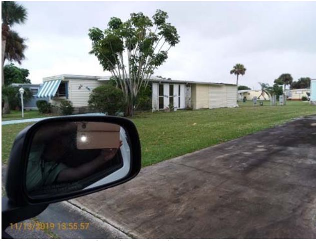
891 Pecan. Roof and gutter damage. Nov 13, 2019
