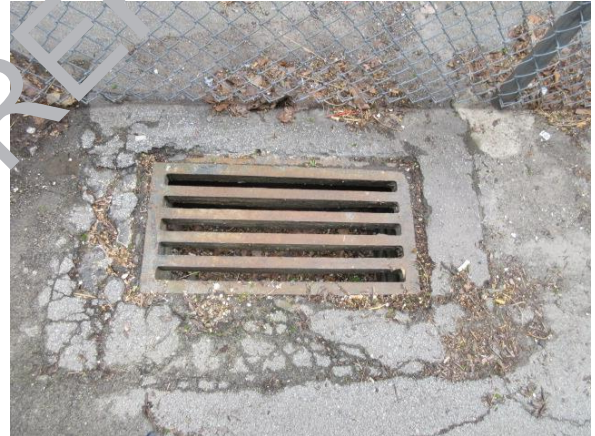
PHOTO #16: PAVEMENT DRAIN
