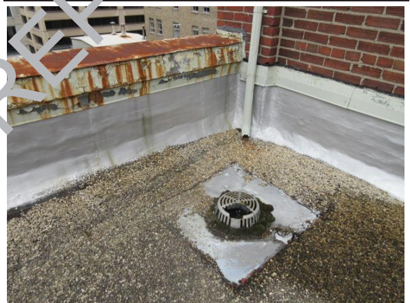
PHOTO #22: ROOF DRAIN
