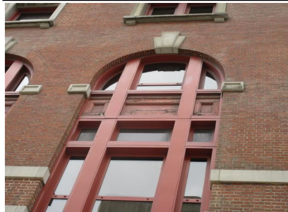
PHOTO #12: SUSPECTED LEAD PAINT
