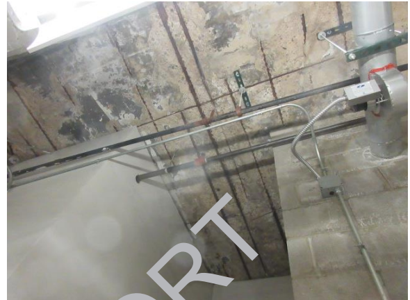
PHOTO #8: FIRST FLOOR SLAB (NOTE EXPOSED REINFORCING STEEL)
