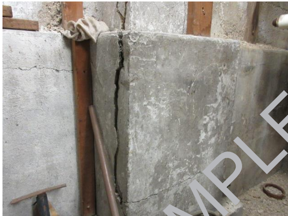
PHOTO #9: COLUMN BASE (NOTE CRACKED CONCRETE)
