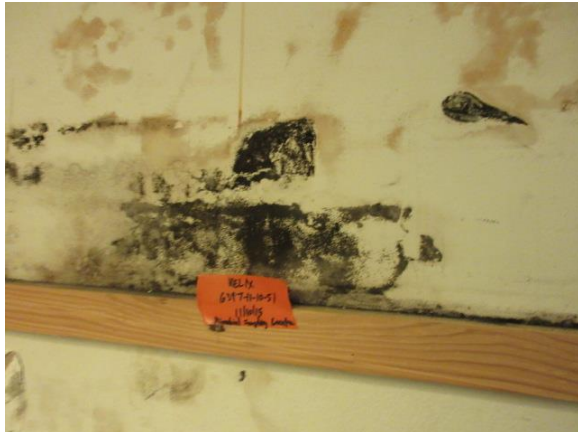
PHOTO #7: EVIDENCE OF MOLD IN BASEMENT
