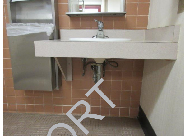
PHOTO #14: ACCESSIBLE LAVATORY (PIPE SHOULD BE INSULATED)
