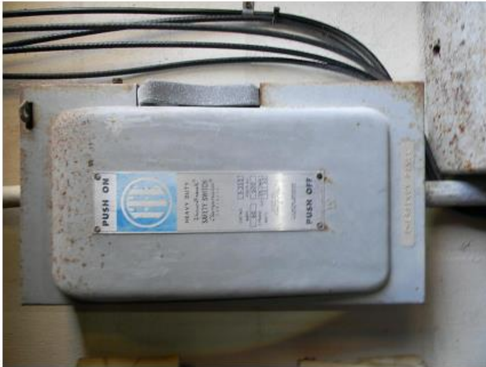
Old Disconnect Switch for Emergency Panel
