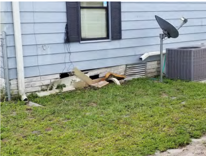
406 Papaya Skirting needs to be replaced / repaired. BBRD ARCC permit required.
