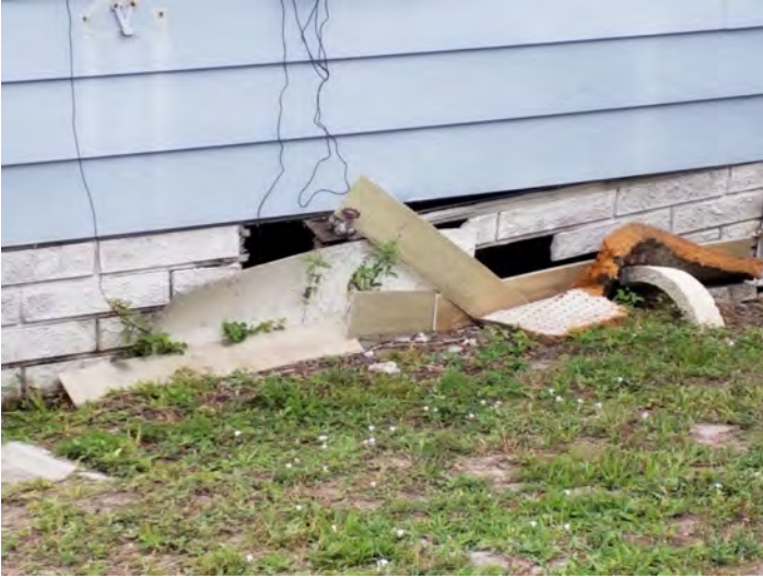
406 Papaya Skirting needs to be replaced / repaired. BBRD ARCC permit required. Jun 06, 2022
