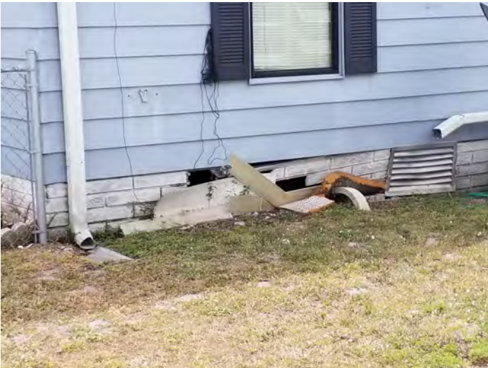
406 Papaya Skirting needs to be replaced / repaired. BBRD ARCC permit required. May 03, 2022
