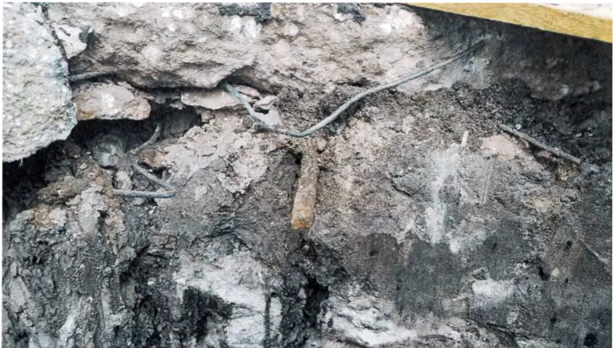
Photo S13 – Test Pit 3 (post-excavation): Existing Cut Tie-Back
