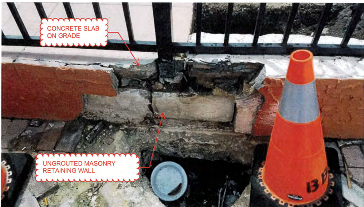
Photo S6 – Test Pit 1B (post-excavation)
