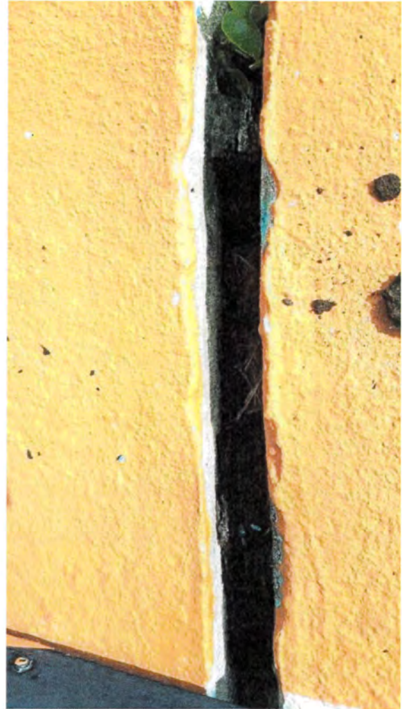
Photo S17 – Existing Joint in Wall Cap
