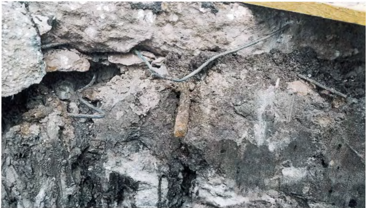
Photo S13 – Test Pit 3 (post-excitation): Existing Cut Tie-Back
