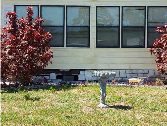
309 avocado Skirting / vent cover needs to be replaced / repaired. 06/02/2023
